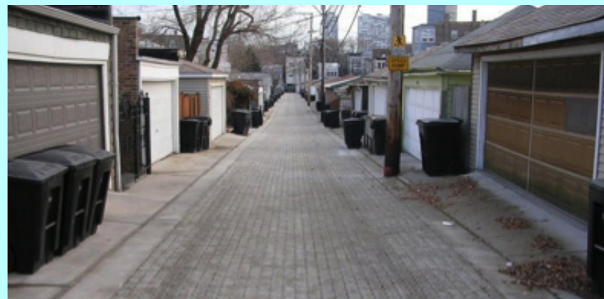
Permeable Pavers and Permeable Concrete Chicago Alleys (Source: Abby Hall, US EPA, p 17)
